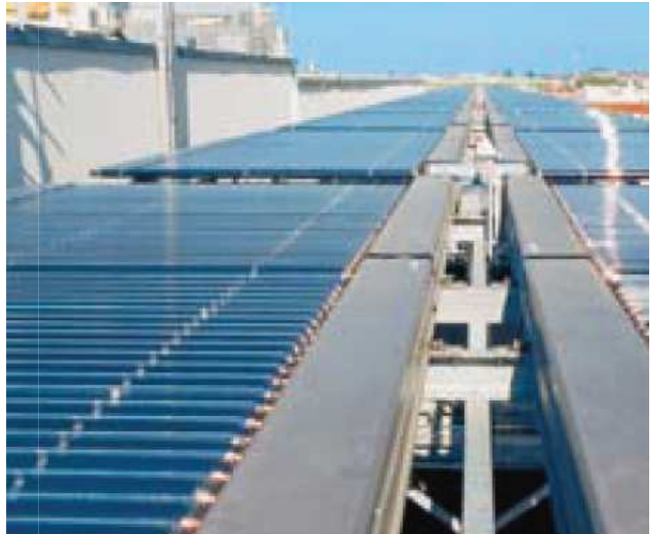
Flat roof installation (horizontally)
