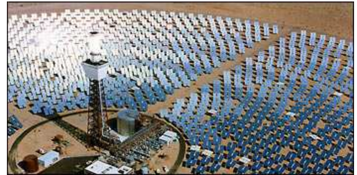
Concentrated solar power
