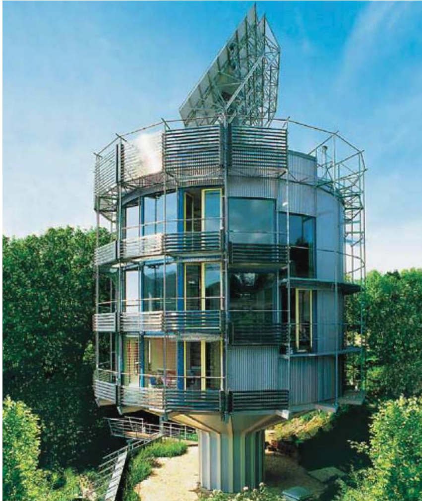
Collectors as a design element of the Heliotropes in Freiburg, Germany.
